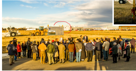
Nov 11, 2007 - Ground Breaking; McDonald Nissan partially circled. Good view of the west end of the casino building. (David Tanaka photo)
